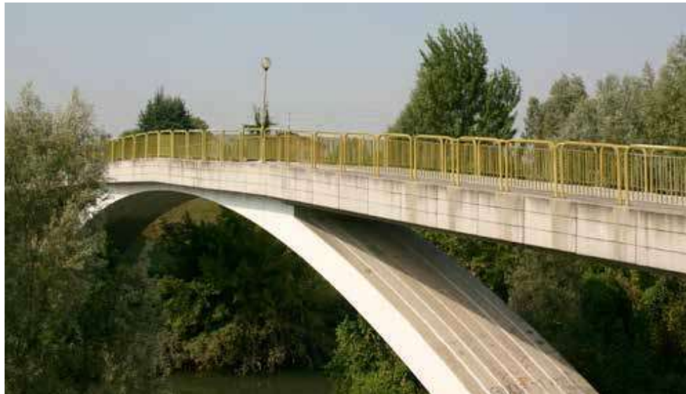
Footbridge over the Bacchiglione River - Padua (Italy)
