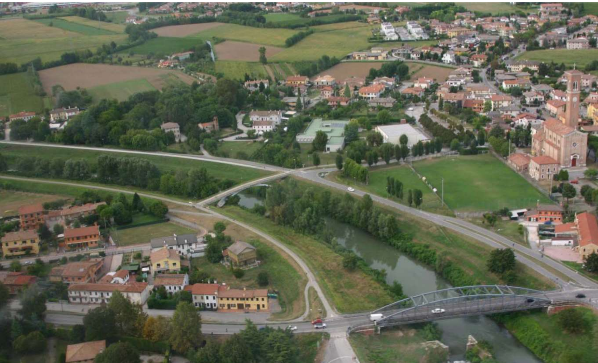
Footbridge over the Bacchiglione River - Padua (Italy)
