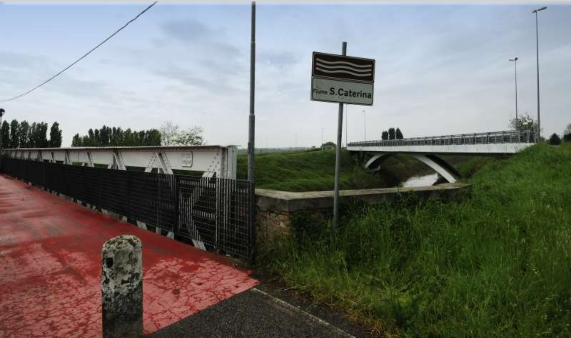
The bridge over the S. Caterina Canal – Padua (Italy)
