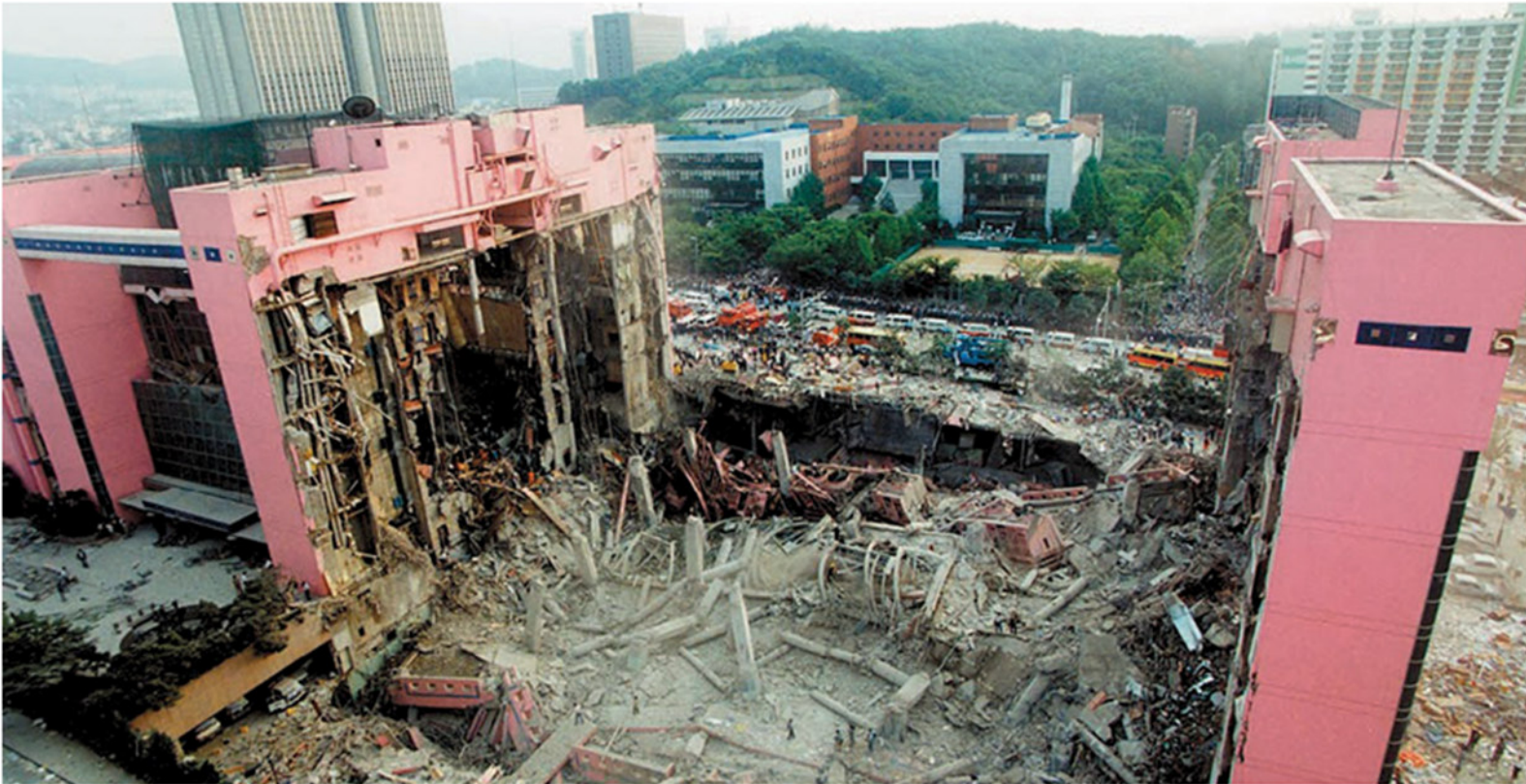
The Sampoong Department Store collapse remains one of the most tragic structural failures in modern history. 5
