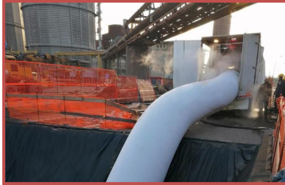
CIPP - Cured in place pipe
